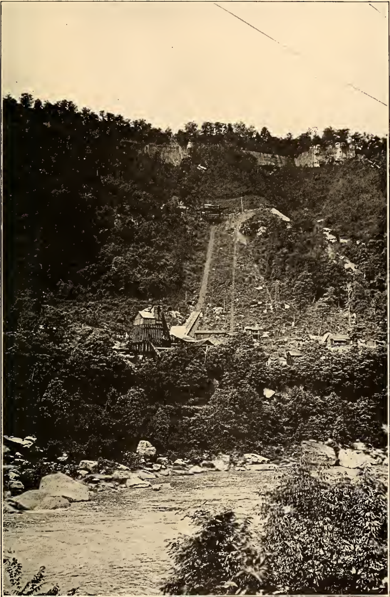
Photo furnished by C. E. Krebs. PLATE XIX.—View showing coal tibble and incline railway to opening in Sewell Coal of Marr Branch Coal Co., on west hillside of New River at Whitney; cliffs of Lower Nuttall Sandstone near sky-line.
